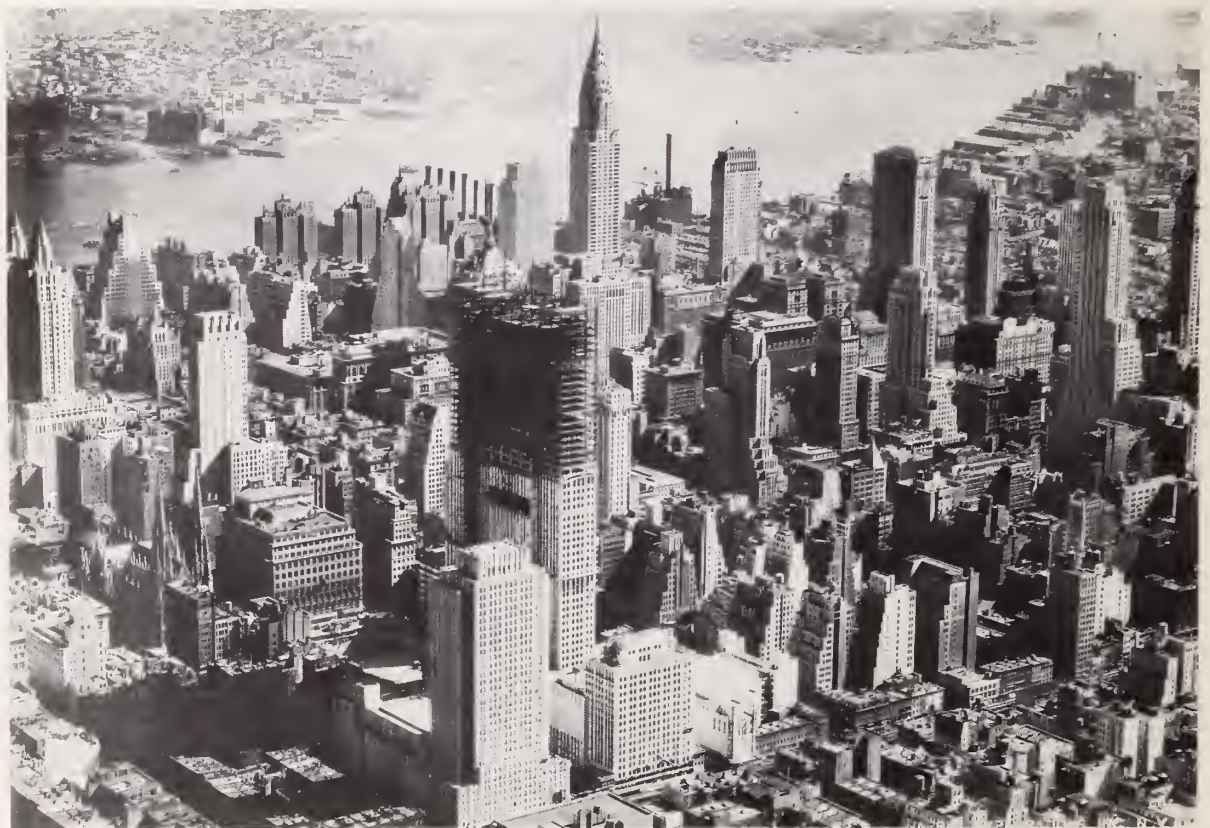
Fig. 30. Aerial view, Rockefeller Center, 1932, looking east across Avenue of Americas.
